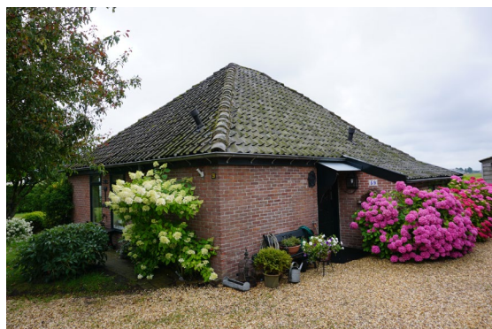
Entree in westgevel
